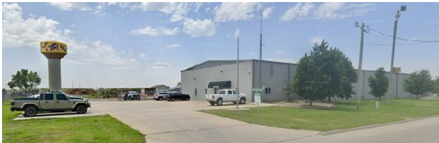
Valley Center Public Works Building
