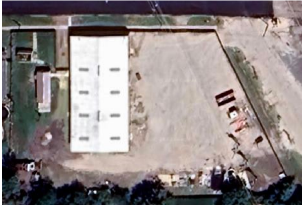
Aerial— Valley Center Public Works Storage Facility
