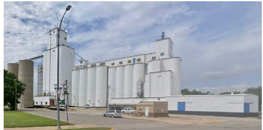
Grain Elevators in Valley Center
