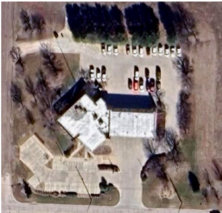
Aerial – Valley Center Public Safety Building
