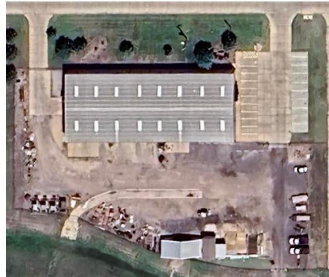
Aerial – Valley Center Public Works Building
