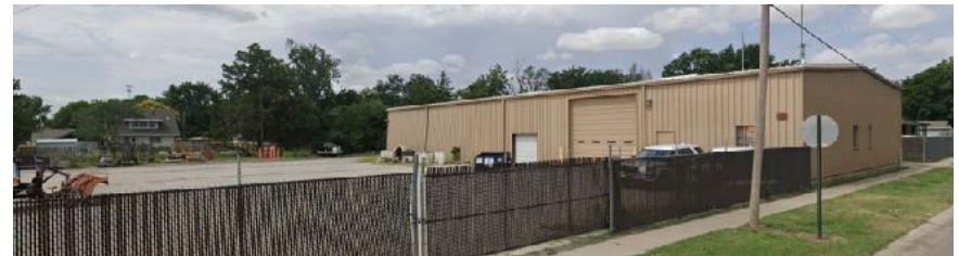
Valley Center Public Works Storage Building—east facade
