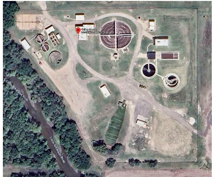
Aerial – Valley Center's Wastewater Treatment plant
