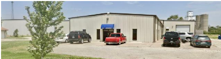
Typical industrial facilities in Valley Center's Industrial Park
