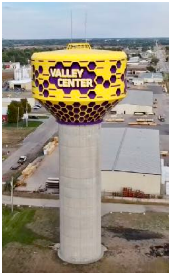
Valley Center water tower
